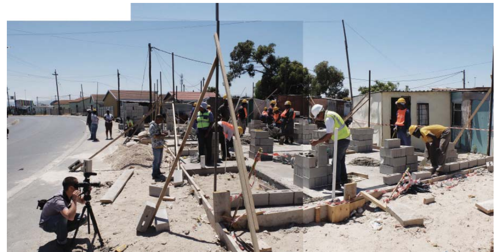
Empower Shack Prototype Housing Under Construction 2016
